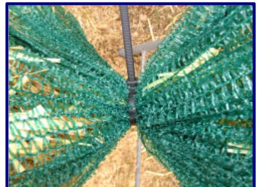
**Step 7:** Cut off the netting at the end of the sausage and tie a knot in the end. Tie about 1.5 m of rope or baler twine around each end.
